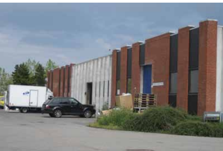
Hammerholmen HBI Light Industrial, Denmark
