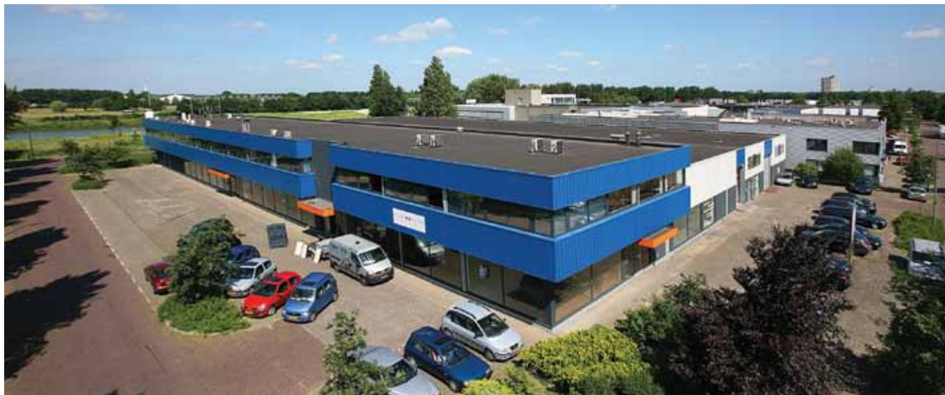
Vlaardingen asset, HBI Light Industrial, Netherlands
